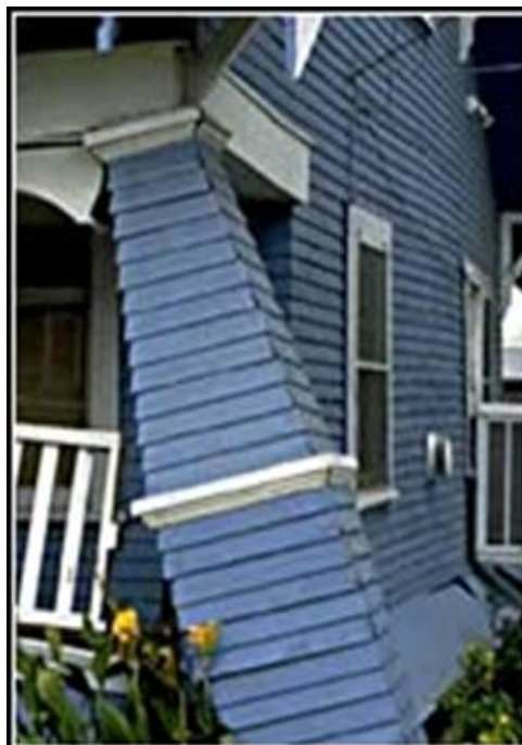
Figure 26: Structural Earthquake Damage
