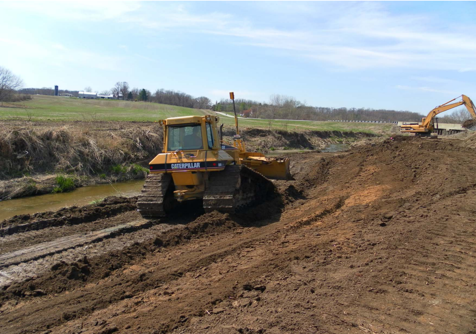
2_stage ditch construction
