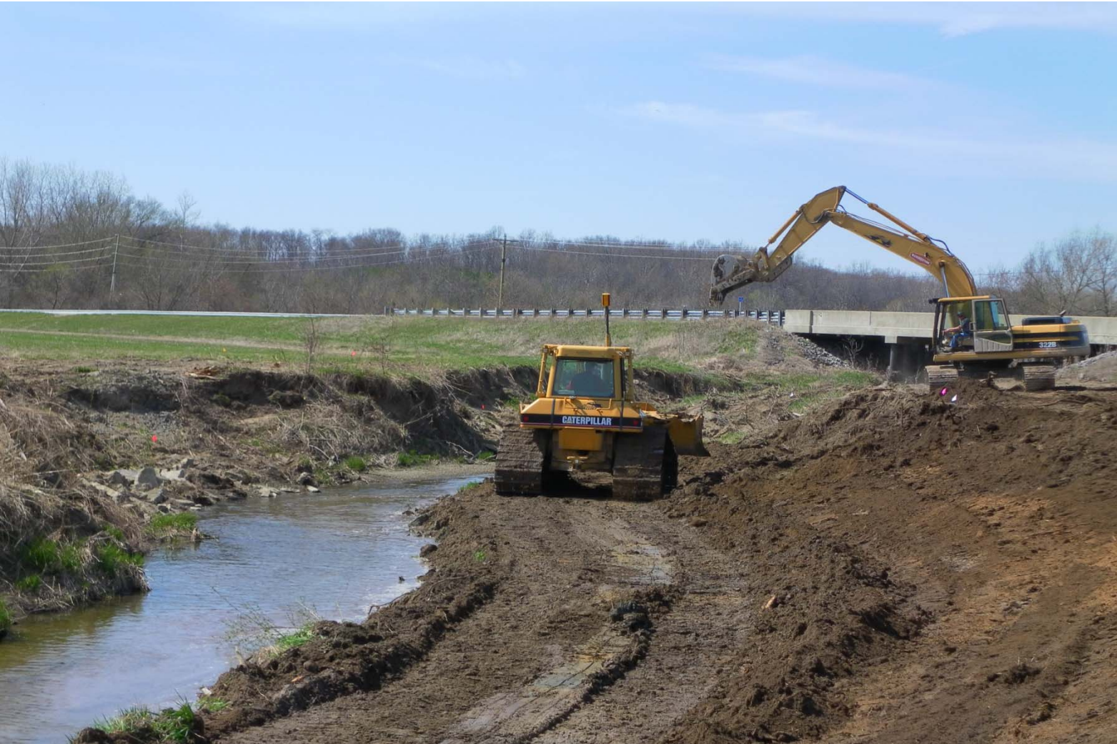
2_stage ditch construction
