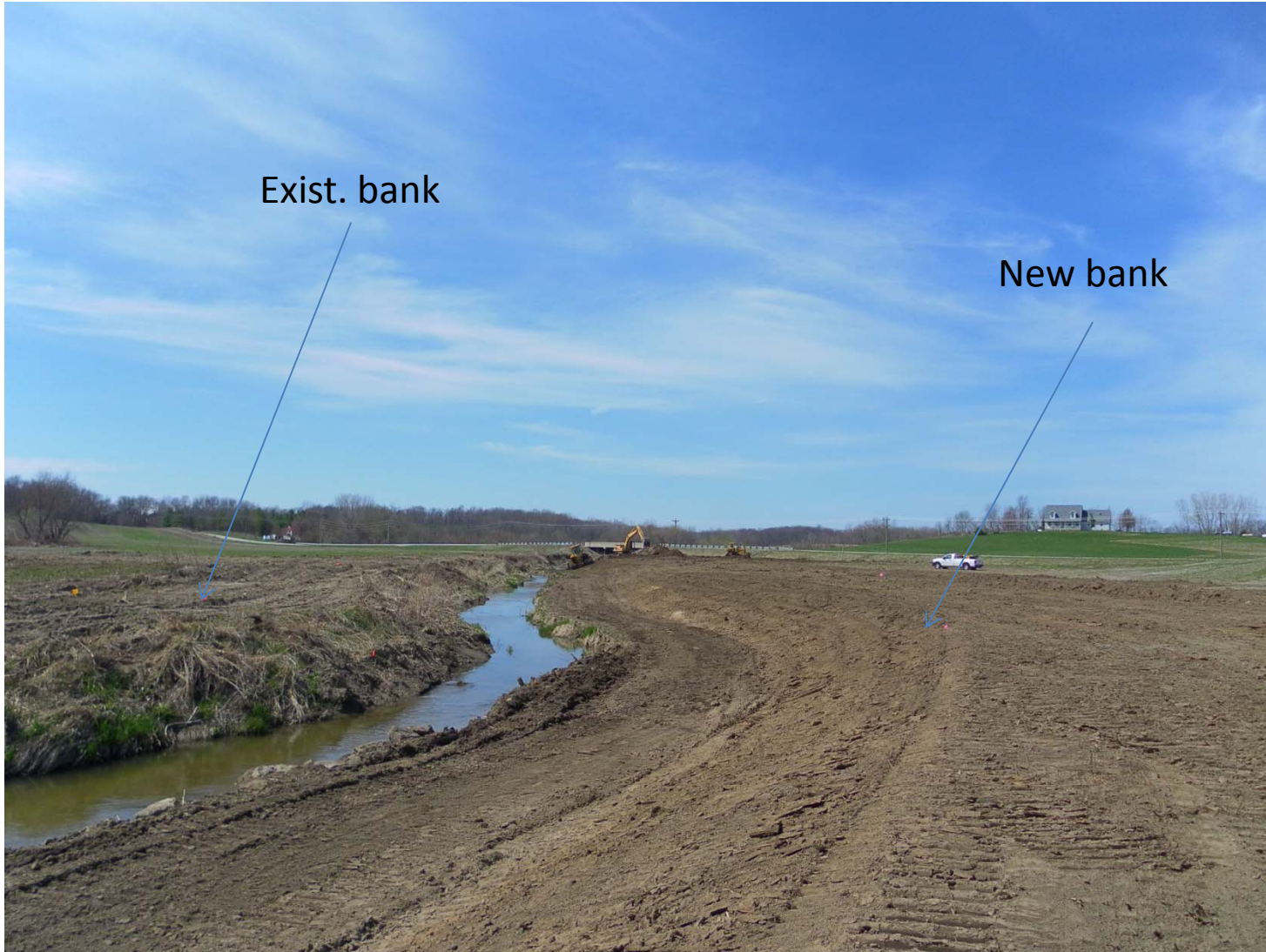
2_stage ditch construction
