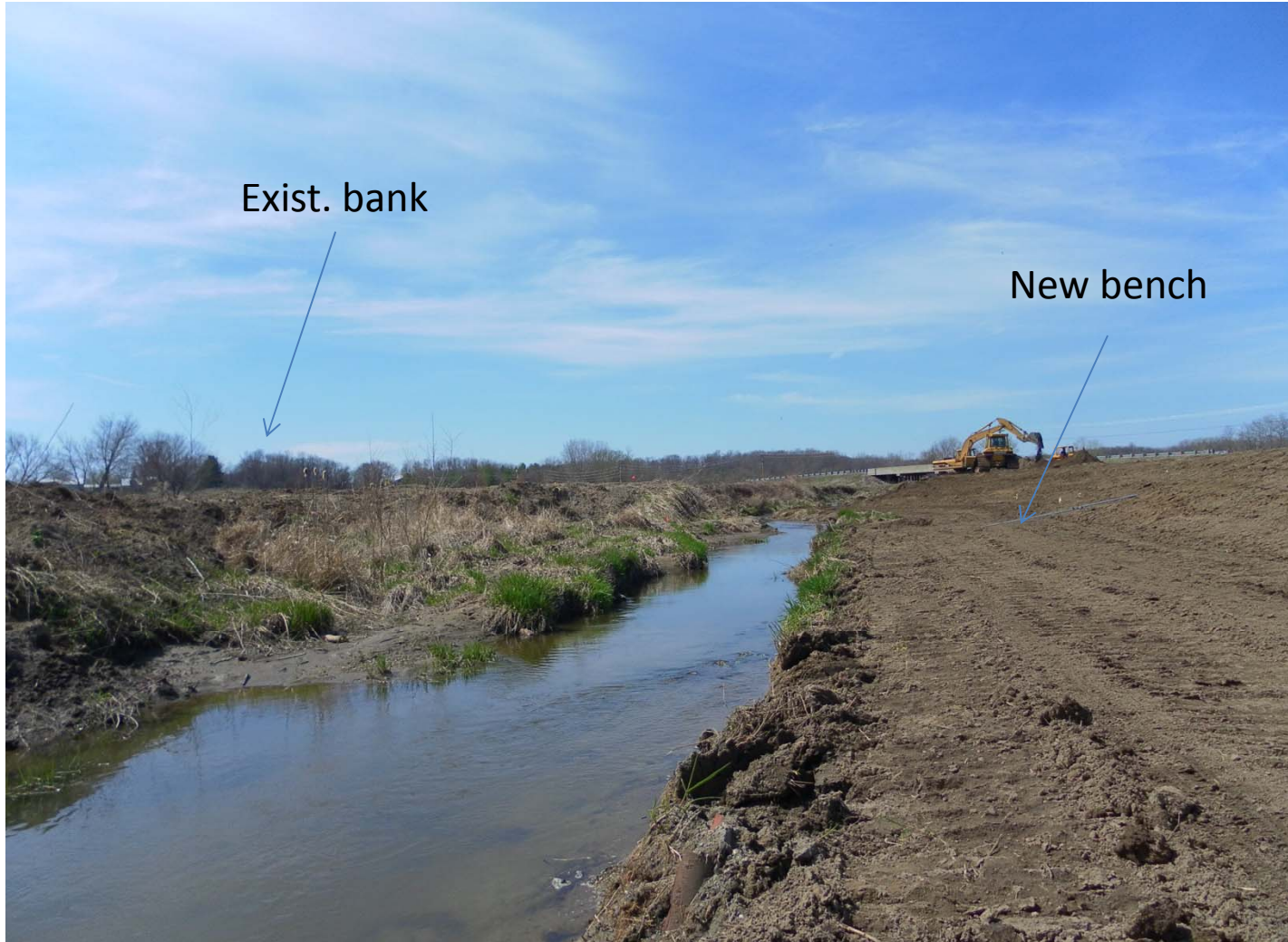
2_stage ditch construction
