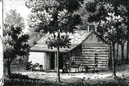
OLD HOME, BUILT 1845.
